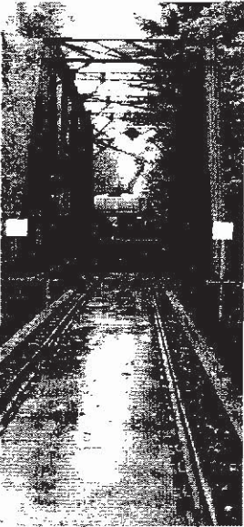
Albany & Eastern Railroad bridge upgrade, a ConnectOregon II project
